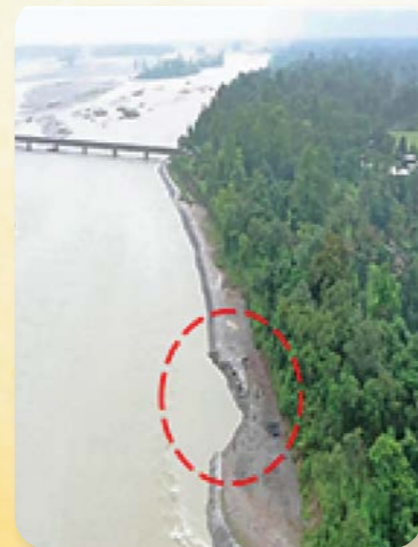
Extensive Damage to Guide Bunds
