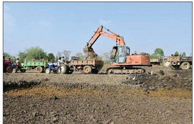
Lake Rejuvenation in progress
